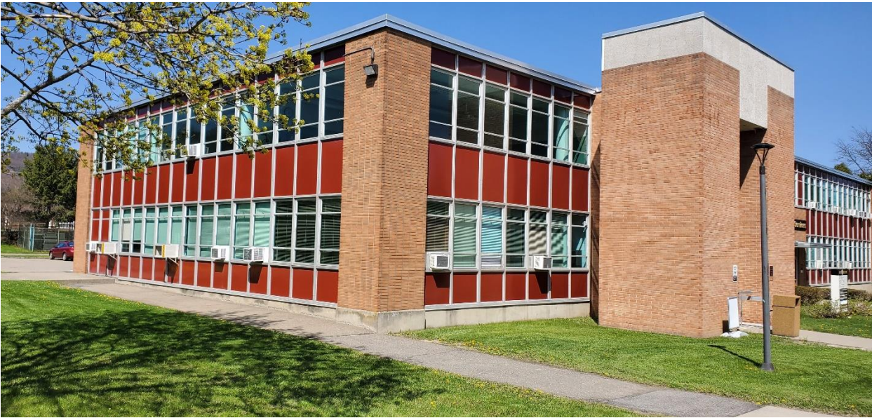
Built in 1956-57, this building at SUNY Broome needs a complete renovation. Window AC units need replacements and are loaded with asbestos, which adds greatly to the renovation costs.
